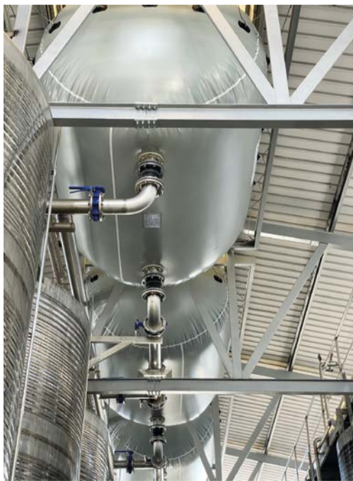
DETAILS IN THE SYSTEM THAT "CAPTURES" AND RE-USES CO 2 PRODUCED DURING THE FERMENTATION PROCESS
